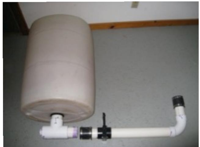
*The entire drain assembly minus the fish tank and hose (left side of 't')*
