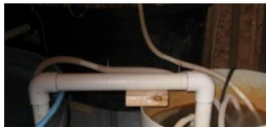
*U-tube used in conjunction with center drain.*
