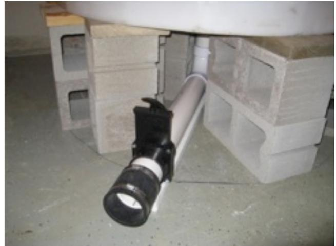
*A view of the drain assembly under a different tank.*
